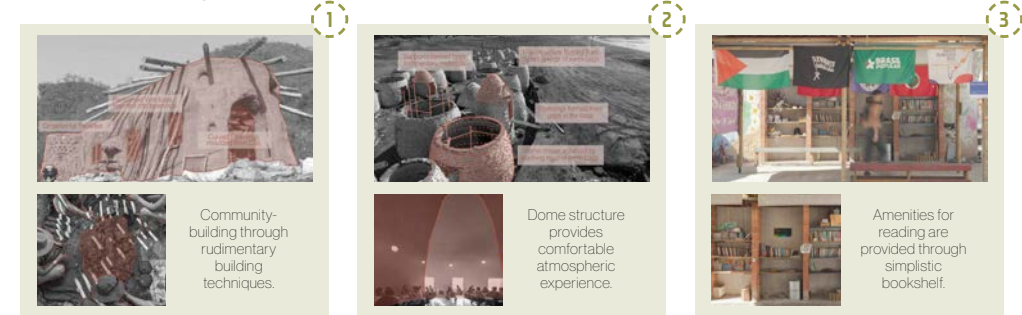
'Tiny Farm Fort' by Tiny Farm Labs - building with cob (clay soil/straw/sand/water) for thick natural walls.
