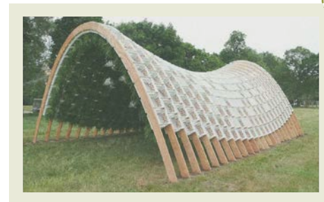
Living Pavilion by Ann Ha and Behrang Behin - a pavilion that uses milk crates as the exterior framework for growing planted surfaces on the interior.
