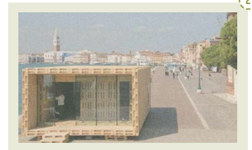
Pallet House by Schnetzer Andreas Claus and Pils Hregor - reuses pallets to create modular, energy efficient and affordable housing for $11 USD per sq. ft.
