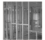
TIMBER CONSTRUCTION FOR PARTITION WALLS FOR STORAGE
