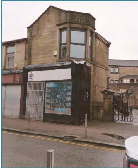
Existing Front View
